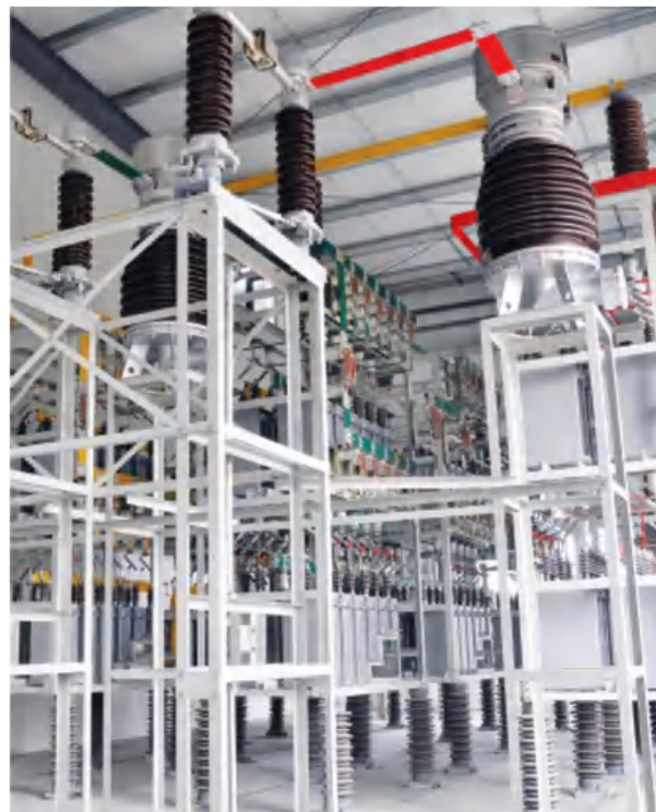
▲电容塔 Capacitance Tower
